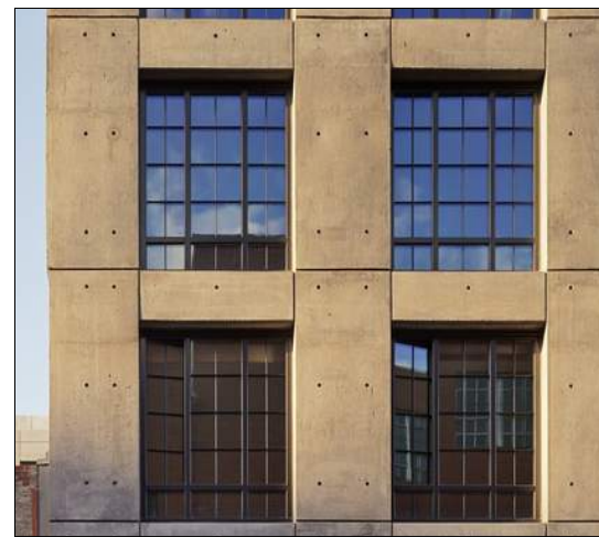
⑫ PRECAST CONCRETE PANELS
