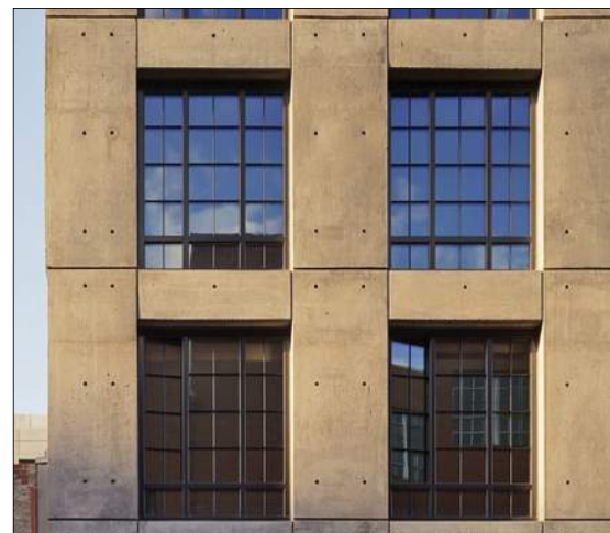
⑫ PRECAST CONCRETE PANEL
